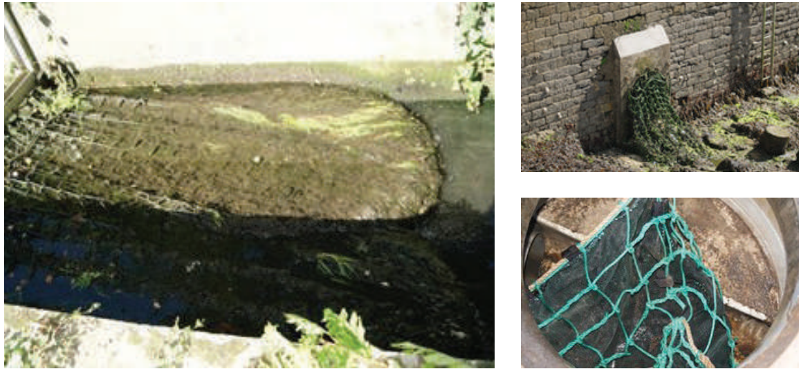
Figure 12: Retention nets in place in Brest Métropole in waterways, rainwater outlets and downspouts (Photos OiEau)
