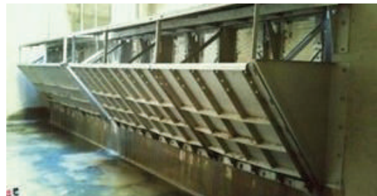
Figure 16: Vertical bar screen. Source/credit: Hydroconcept
