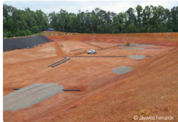
Sanitary landfill under construction , Sri Lanka
