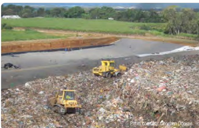
A transfer station in Mauritius
