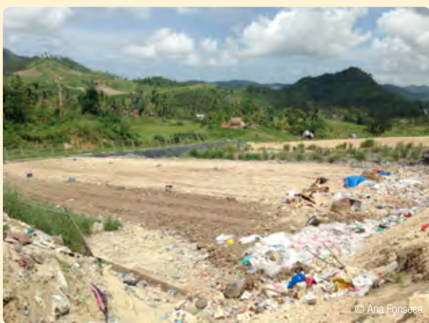
Active cell partially managed: waste compaction, daily cover and vents in place –during UNDP WMC intervention
