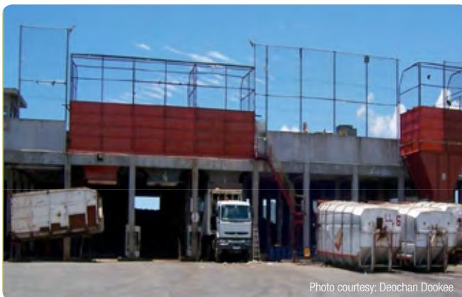
A transfer station in Mauritius
