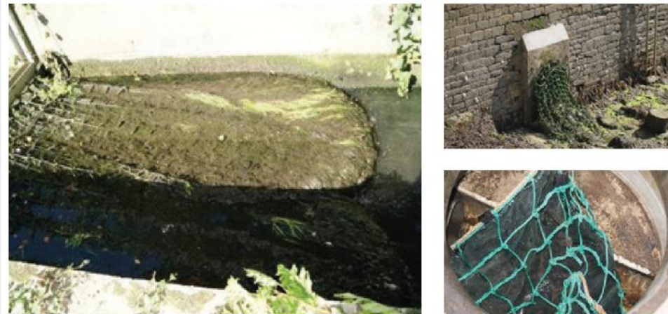
Retention nets in place in Brest Métropole in waterways, rainwater outlets and downspouts (Photos OiEau)
